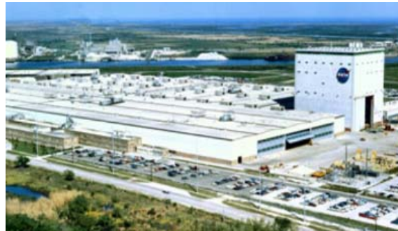
Michoud Assembly Facility New Orleans, LA Project In-Progress by Vanguard Contractors $57,855,287.00
