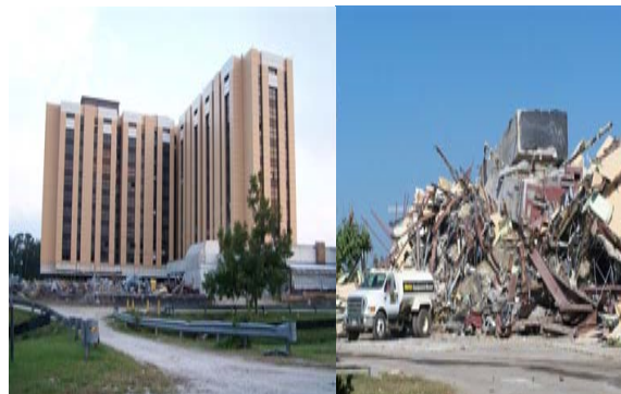
Armed Services Retirement Home Gulfport, MS Project Completed by Ma-Chis LCITE $7,706,856.00
